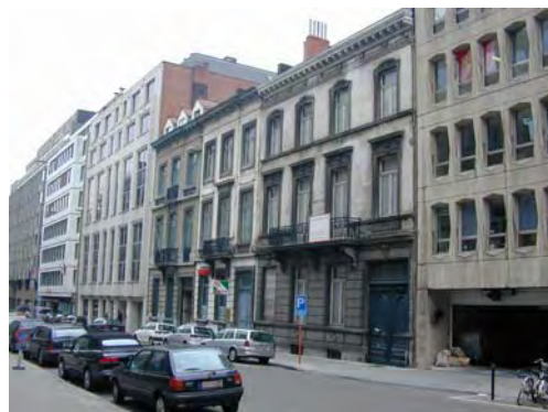
Before & after renovation
