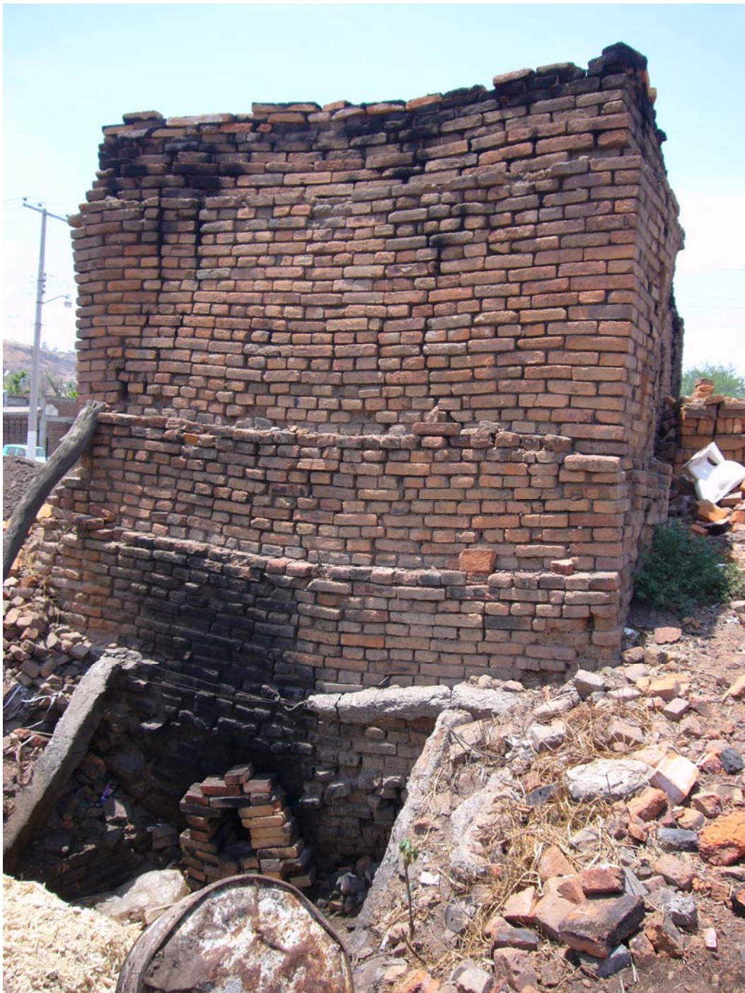
Photo 2: Brick 1. Stationary kiln with underground firing
