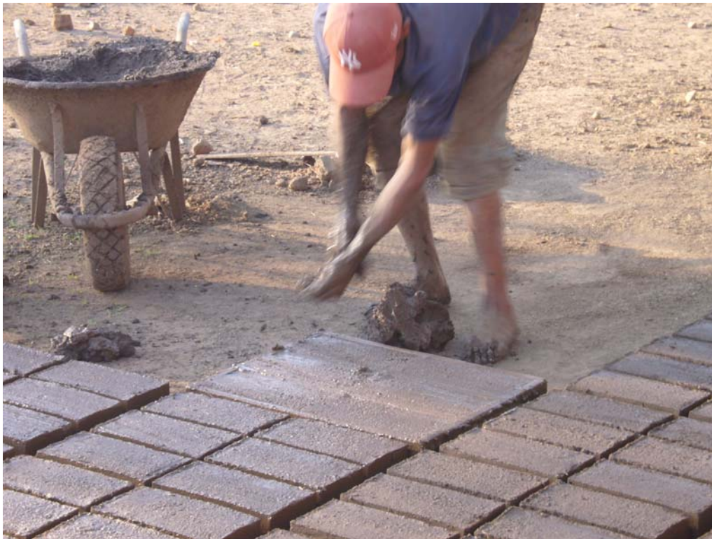
Photo 12: Brick 5. Manual brick making
