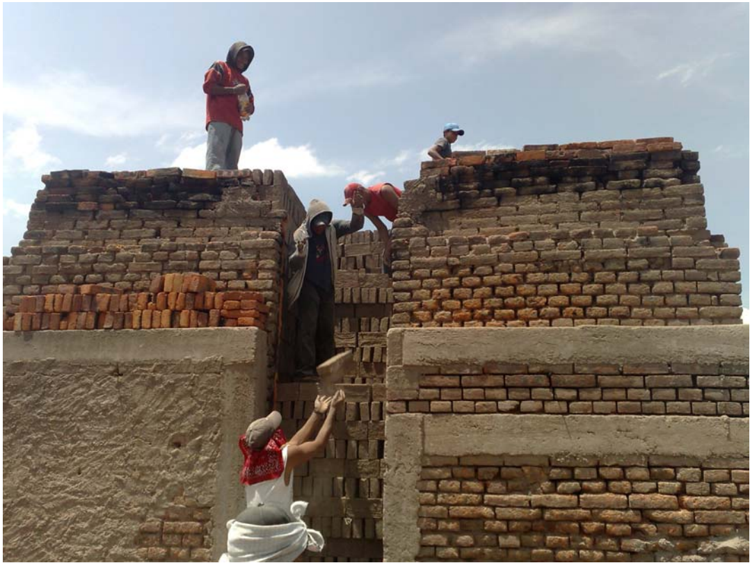
Photo 4: Charging of a stationary kiln with raw bricks
