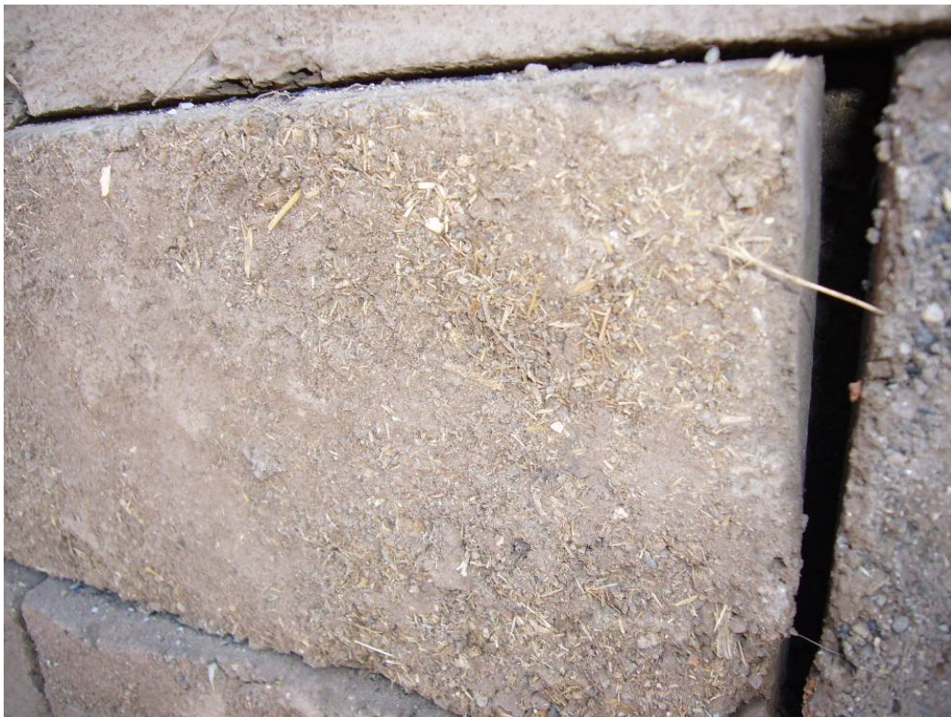
Photo 18: Brick 5. Raw bricks made of dung and clay
