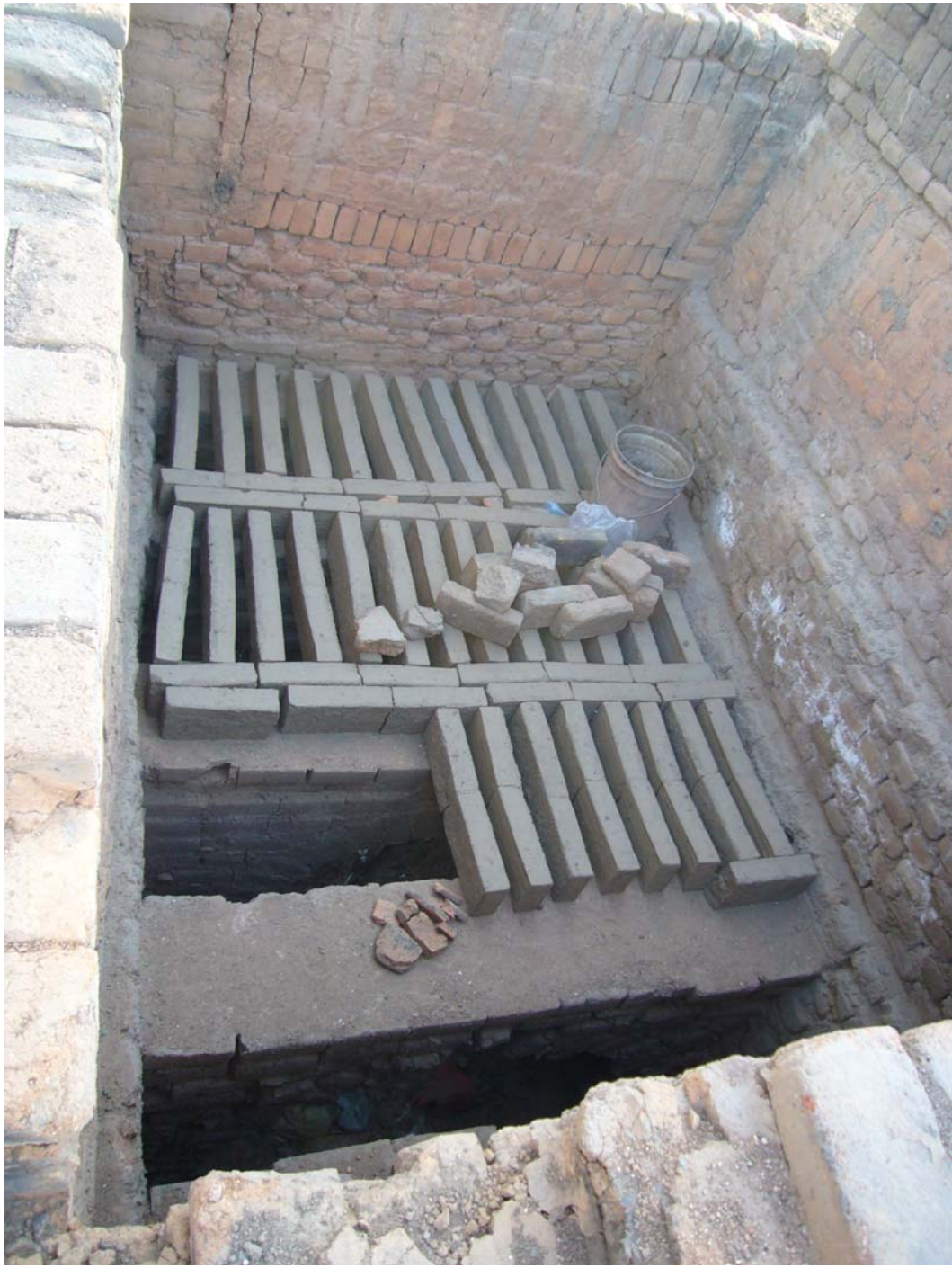
Photo 3: Inside view into an empty stationary kiln
