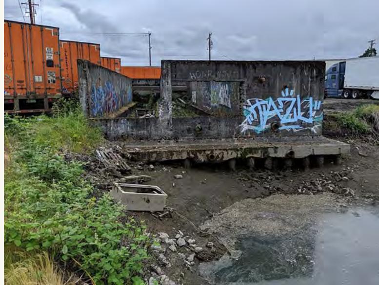
FIGURE 10. OUTFALL 254 ON THE WHEELER-OSGOOD WATERWAY DISCHARGES UNTREATED STORMWATER INTO THE PUGET SOUND.
