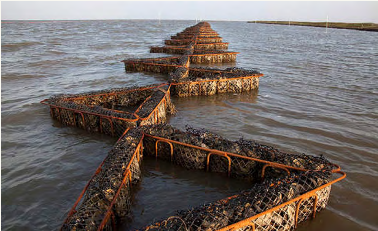
FIGURE 6. ENGINEERED OYSTER REEFS REPLACE FUNCTIONS OF NATURAL OYSTER REEFS.
