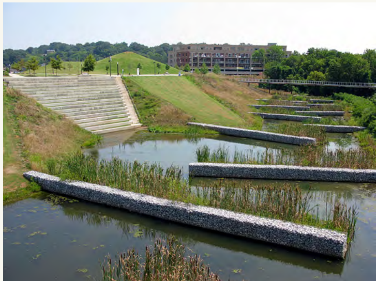
FIGURE 11. EXAMPLE OF ENGINEERED WETLAND
