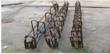
Fig.4.1. Slab contraction joints
