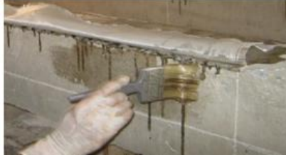
Fig.4.1. Application of epoxy and hardener on beam.
