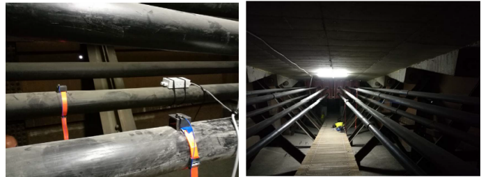
Fig. 1. Monitoring system installation: (1) Plan view of the monitored highway viaduct. (2) MEMS accelerometers installed on the external steel tendons. (3) External prestressing tendons.
