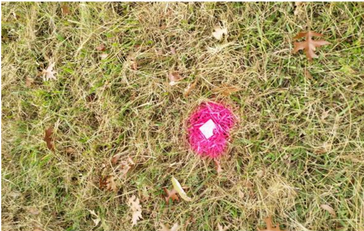
Figure 3. 4: Confirmed marked point free from utilities
