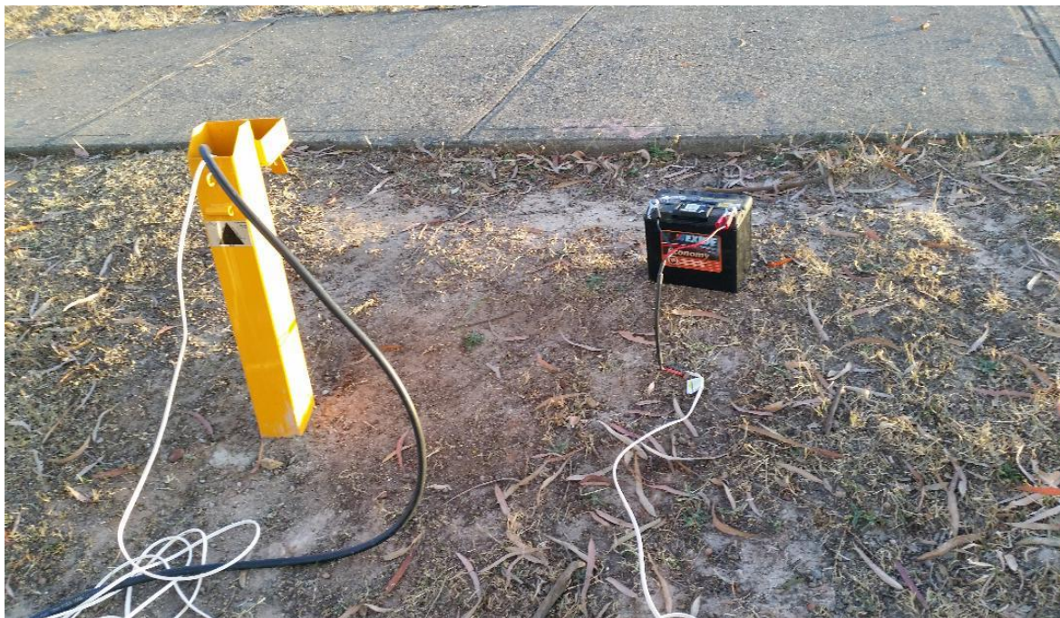
Figure 3. 7: Bore development with a twister pump
