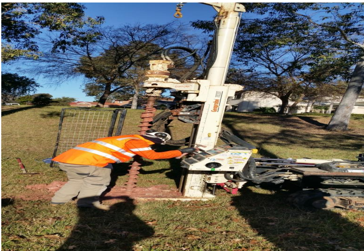
Figure 3. 6: Sectional flight auger drilling
