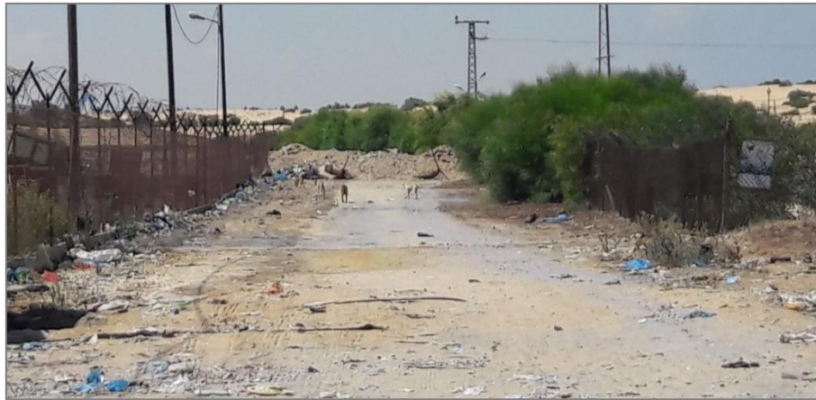
Figure 26. Access Road to Rafah transfer station site
