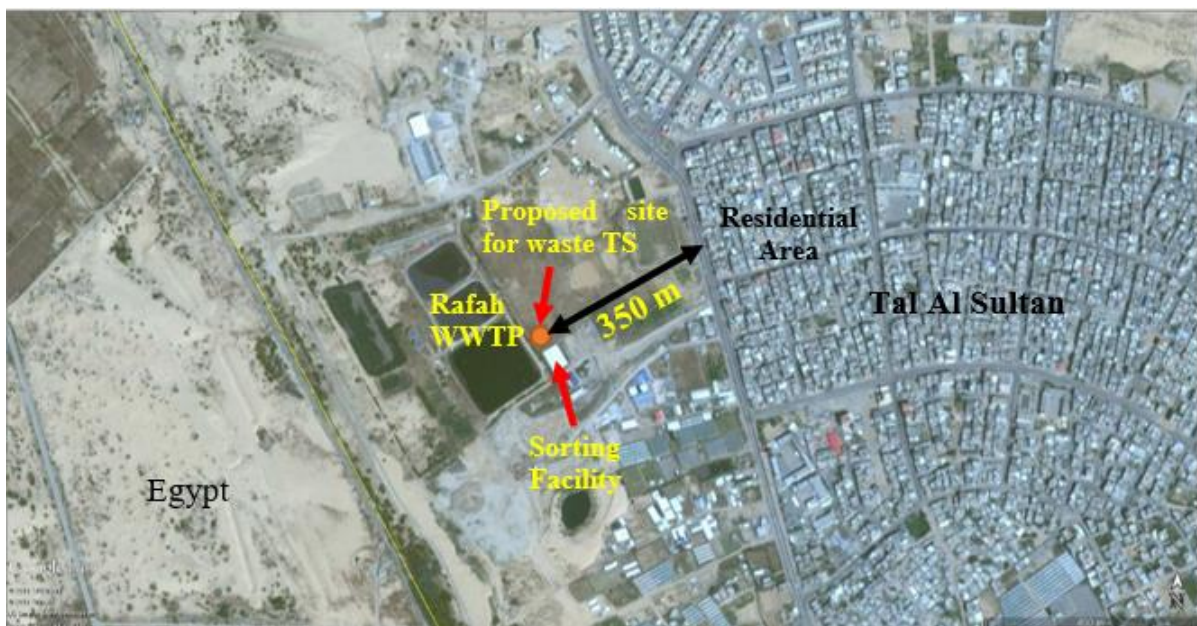
Figure 12. Location of Rafah Transfer Station and the surrounding environment
