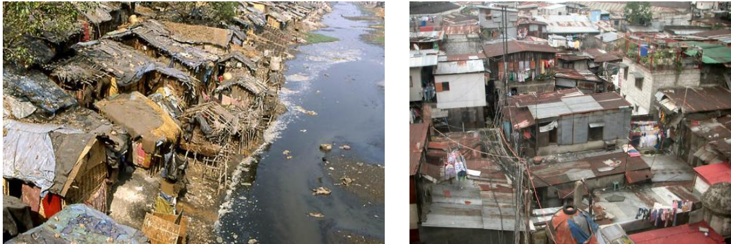
Figure 2.2 and 2.3 Poor structures of housing inside slums. Source: (fotservis.typepad.com,Mother India : Calcutta ,Varanasi)
