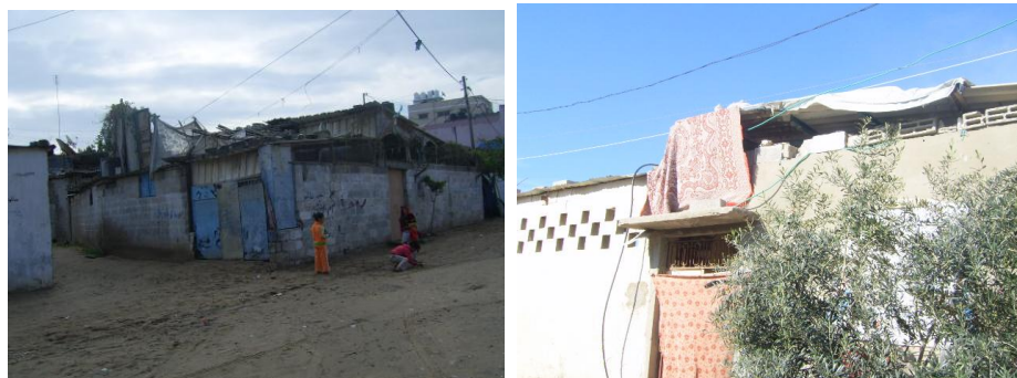
Figure 3.5 Different building materials inside Gaza slums, near Al naser area
