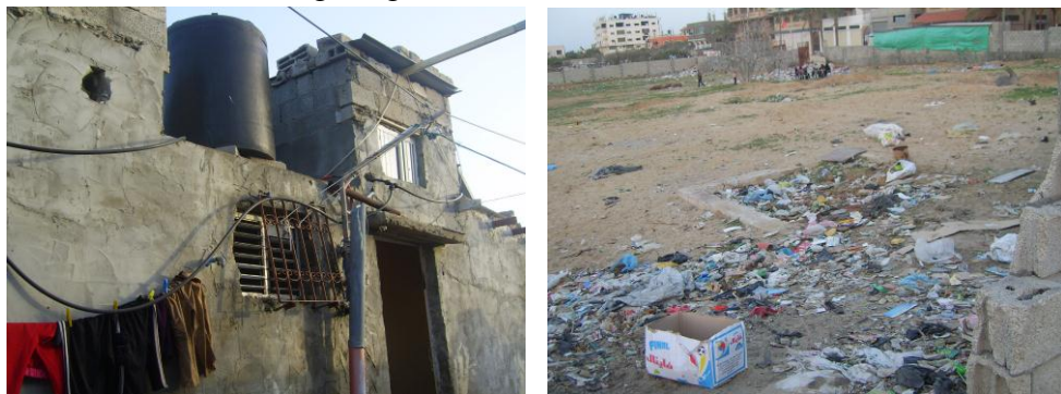
Figure 5.18 lack of services
