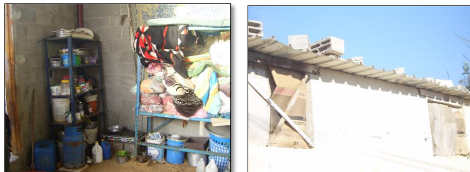
Figure 3.6 Bad conditions of slums buildings. Gaza slums
