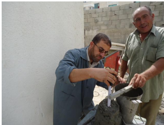
Figure 5.2: Slump level measurement
