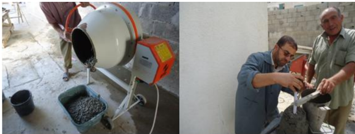
Figure C3: Specimens, Testing ( slump measurements)
