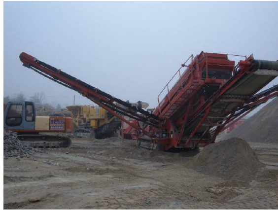
Figure 2.1a: Crusher used to produce RAC at the ready mix concrete plant
