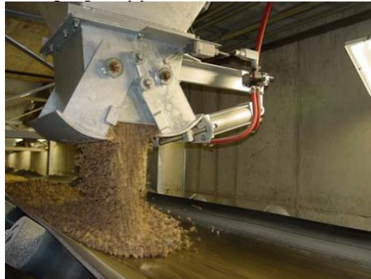
Figure (5.3): Charging Hopper Feed Gates.
