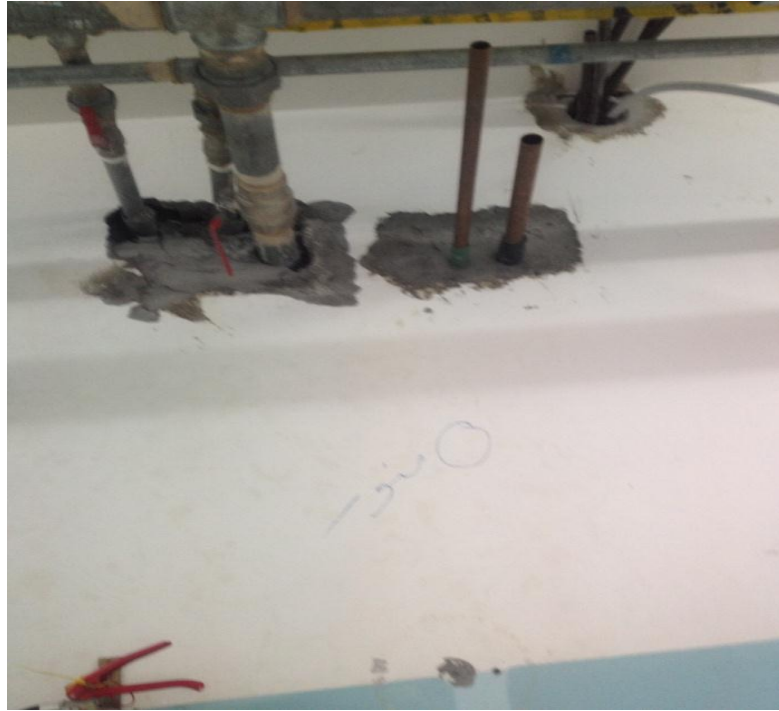
Figure 4.17 Changing water networks
