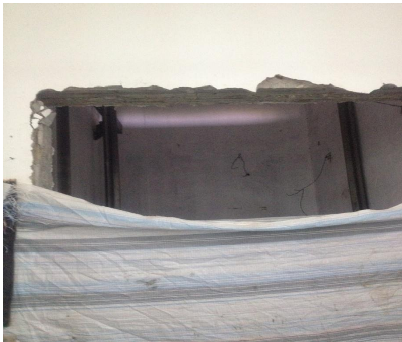
Figure 4.16 Installing new elevator
