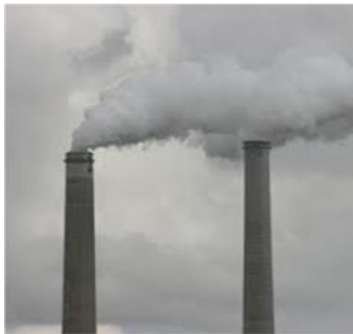
Figure(2.1): Power plant stacks
