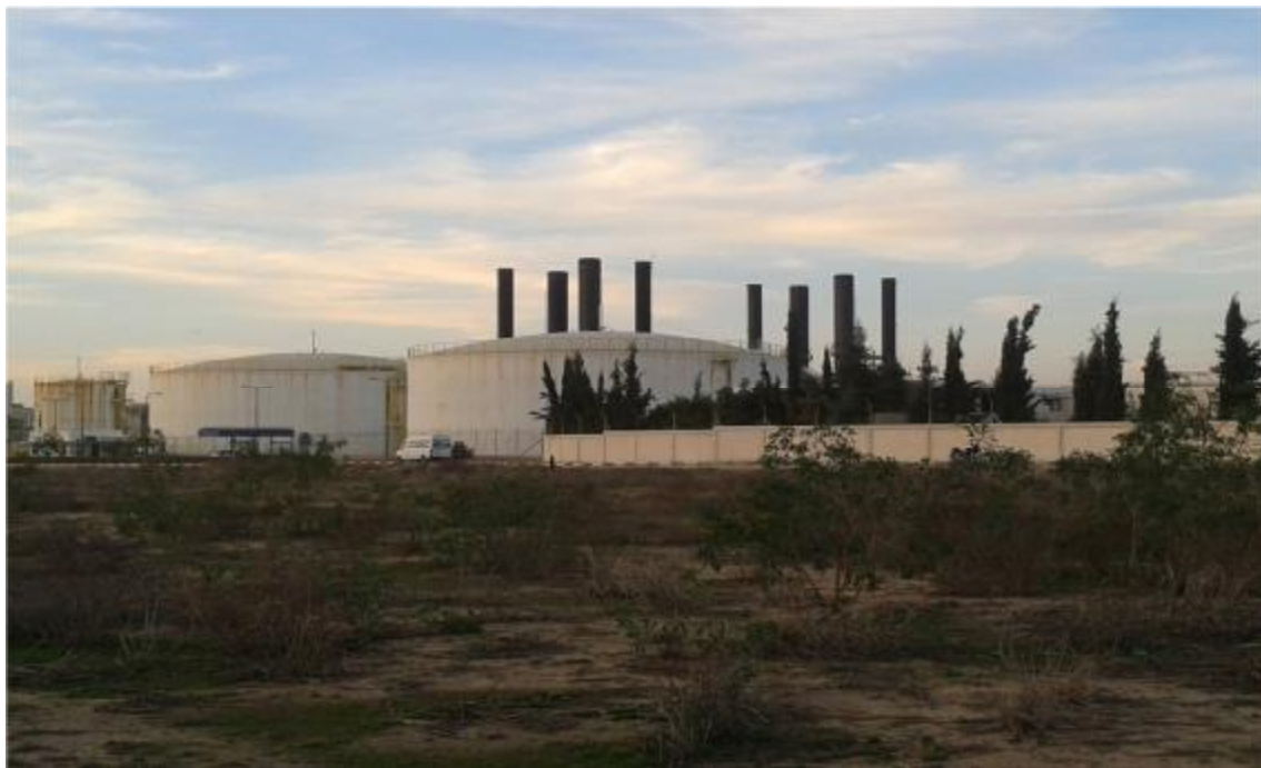
Figure (3.3): Gaza power plant
