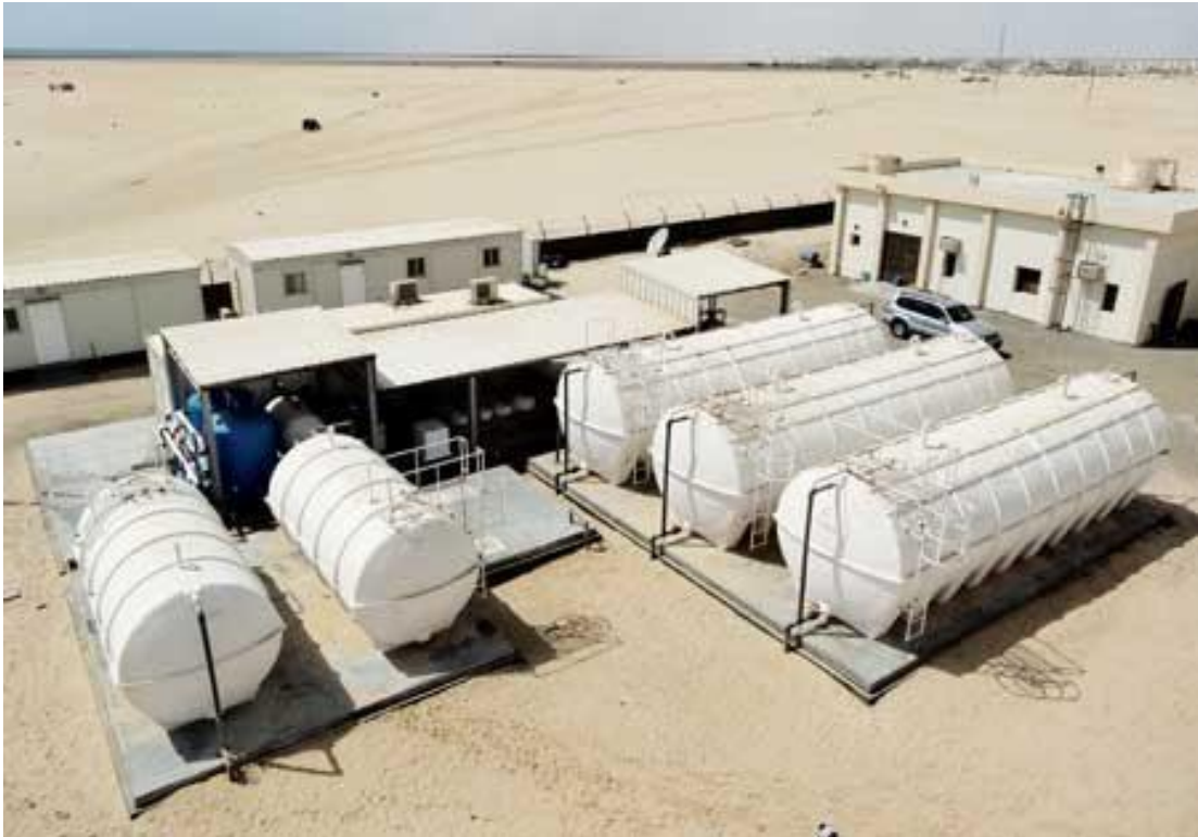
Figure (2.5): Al Najdah desalination plant (200 m 3 /day) at Al Najdah in Oman. (Nicoll, 2013)
