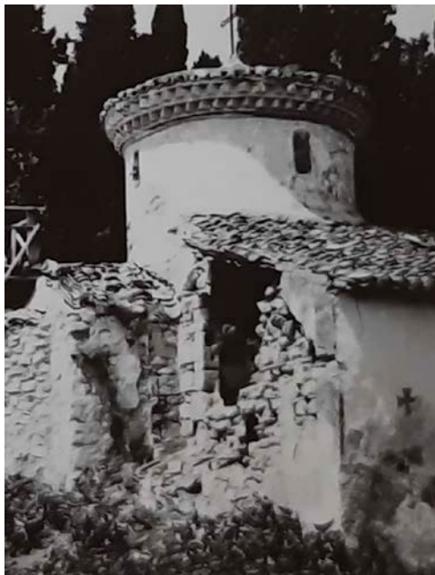
Figure III-5.3 A view of the collapsed apsidal area at the end of the Sixties. The exterior walls and the drum were still plastered. [Courtesy: NICH]
