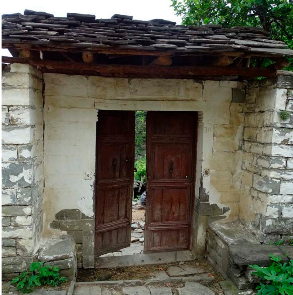
Figure I-4.1.14 A sofat as a transition place between the public and the private dimension of living.
