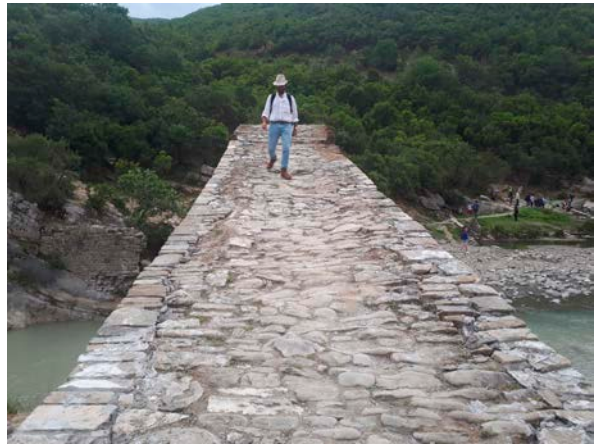
Figure I-5.1.4 – The roadway of the bridge.
