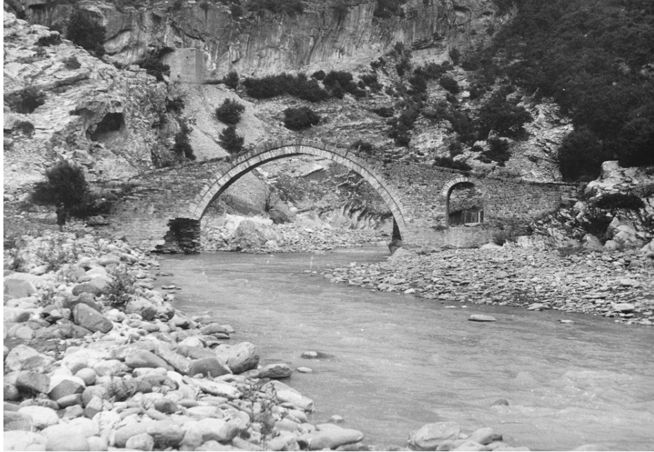
Figure I-5.1.1 View of the Katiu Bridge before the restoration works in 1982 showing the damage suffered by the left abutment (looking upstream) during World War II. [Courtesy: Municipality of Përmet]
