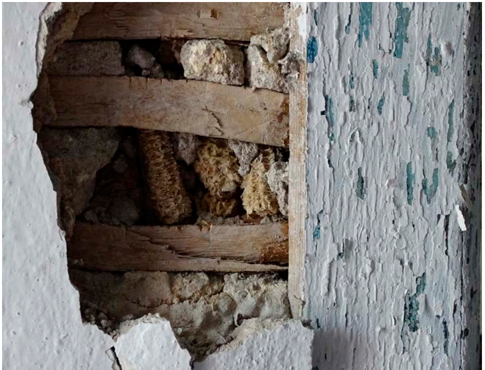
Figure II-4.9. – Trusses in a house of Vrith.
