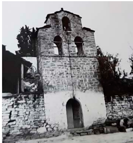
Figure I-5.2.2 The church before the 1982 restoration campaign. Left: View from north- east (with the added volume still present). Right: The XIX Century belfry now demolished. [Courtesy: NICH]
