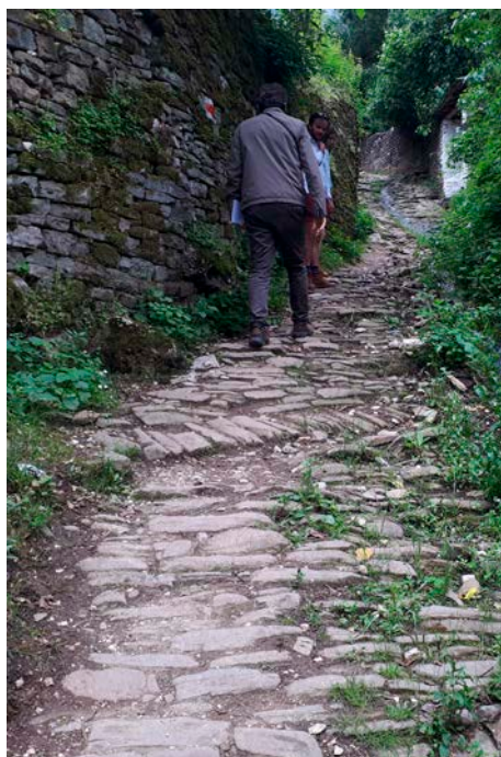
Figure I-2.6 – Leusë. A traditional pavement in kalldrëm.
