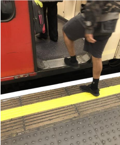
Photograph 4. Gap and step to enter the underground in London
