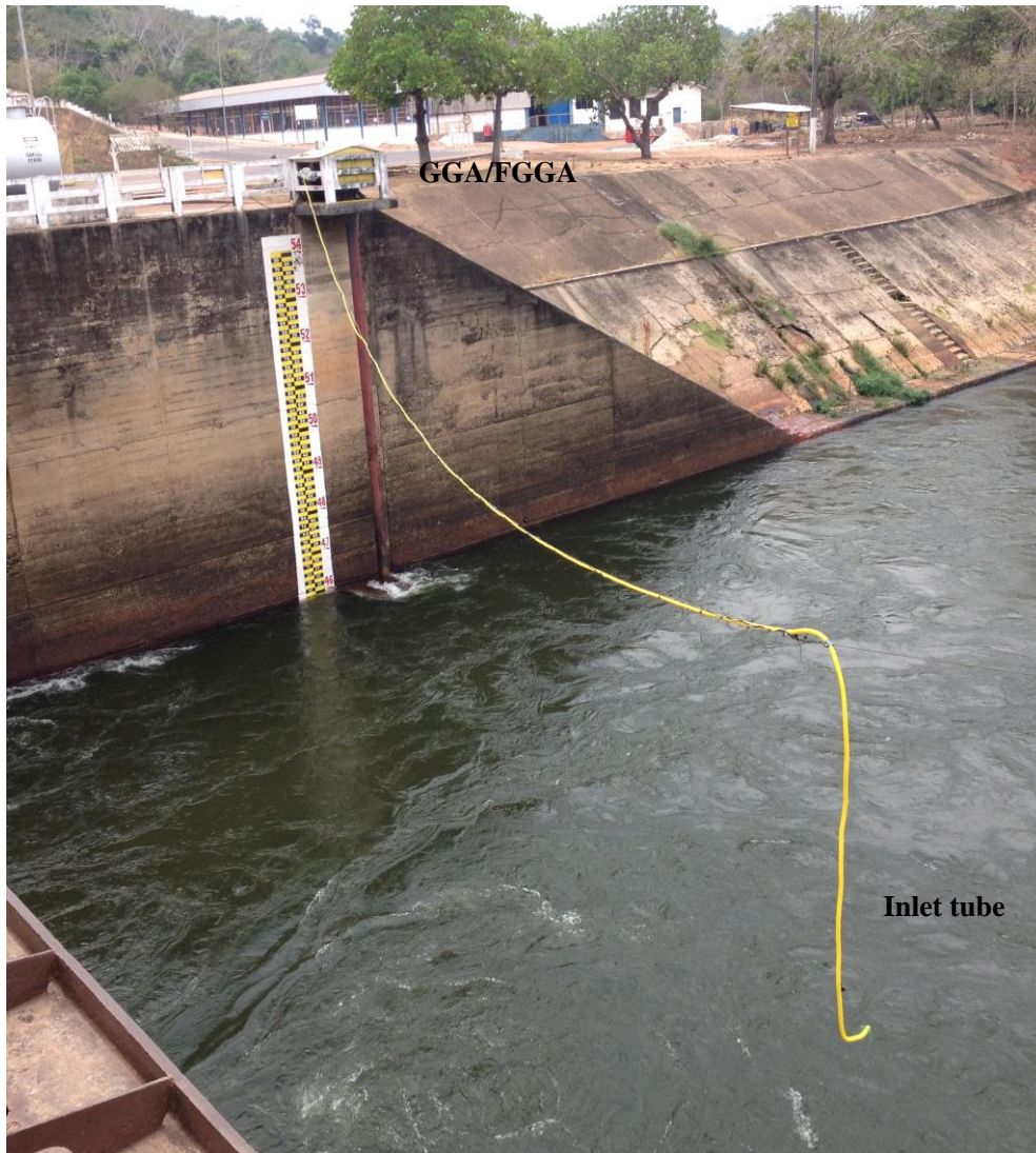
Figure 3. Location of collection of CO 2 and CH 4 samples downstream of the hydroelectric plant. GGA / FGGA (top) and position of inlet tube (below) that collects air samples at about 4 m from the water surface.
