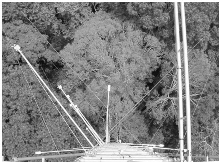
Figure 2. Profile of the nine anemometers installed in the Jarú Reserve micrometeorological tower.
