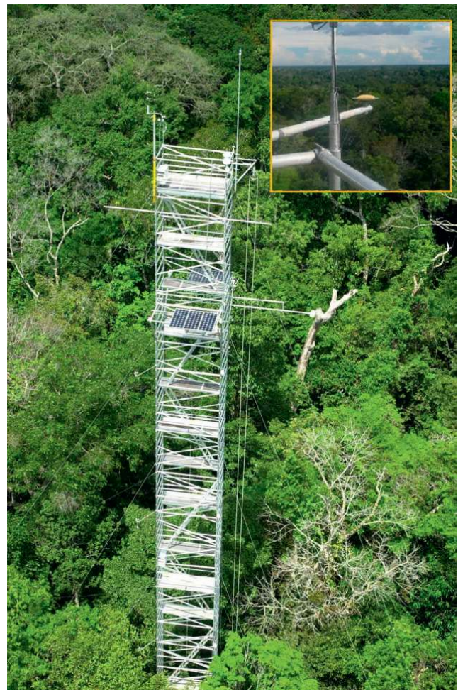
FIG. 1. The 55-m LBA meteorological flux tower K34, located in Amazon rain forest 60 km northwest of Manaus, Amazonas, Brazil. Photo (lower left) was taken prior to placement of any meteorological and flux equipment. Tower extends approximately 15 m above forest canopy. Yellow GNSS antenna (RBDC) on 2-m aluminum tube extends from the side of the tower (inset photo).
