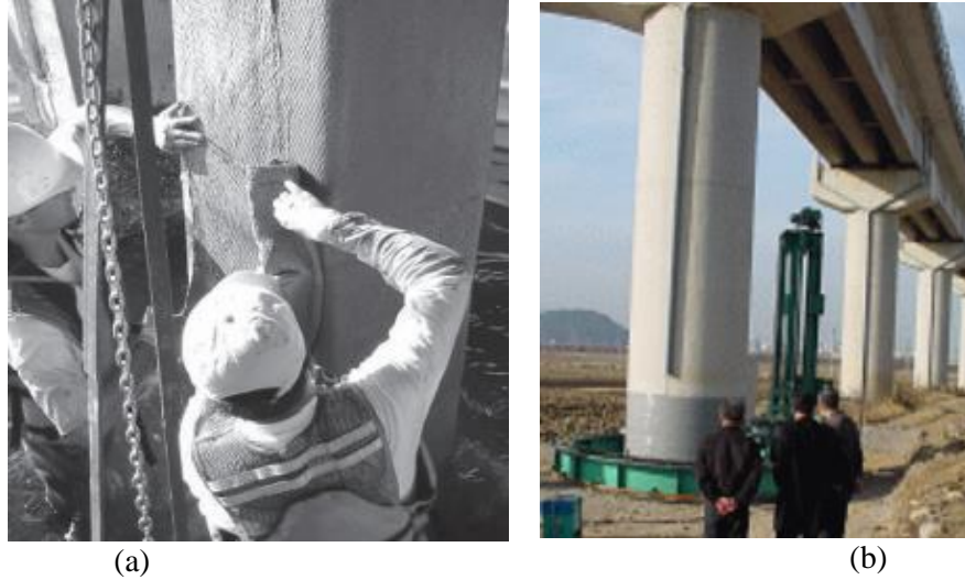
Figure 17. Repaired piers using a) manually (Gandy bridge) [36] b) automatically wrapping (Seomjin bridge) [24]. A single column fitting image.
