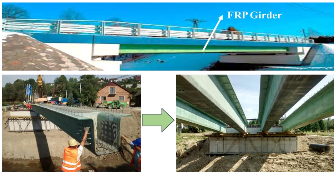
Figure 13. Application of FRP girders for Com-bridge in Poland [87][89]. A 1.5 column fitting image.
