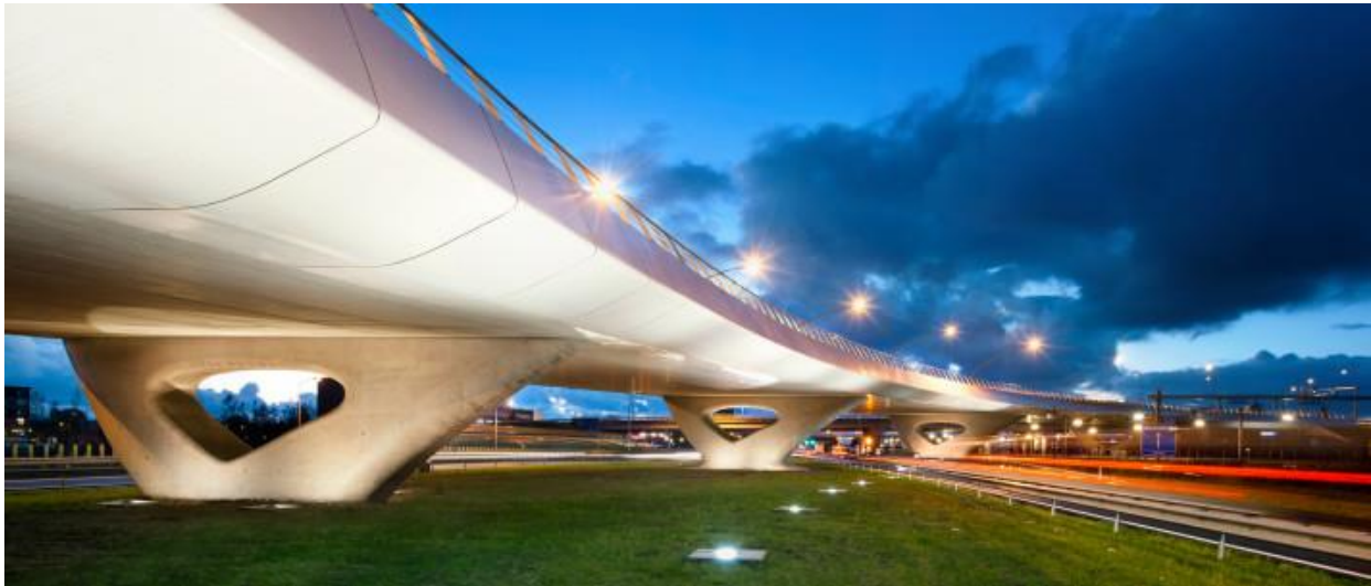
Figure 1. Fly-over Waarderpolder bridge in Netherland with FRP edge elements [10]. A single column fitting image.
