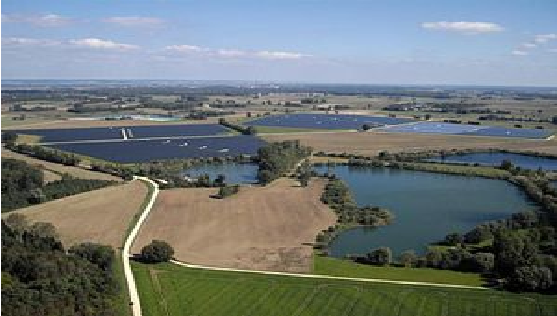
Figure 1.2. The 25.7 MW Lauingen Energy Park in Bavarian Swabia, Germany.
