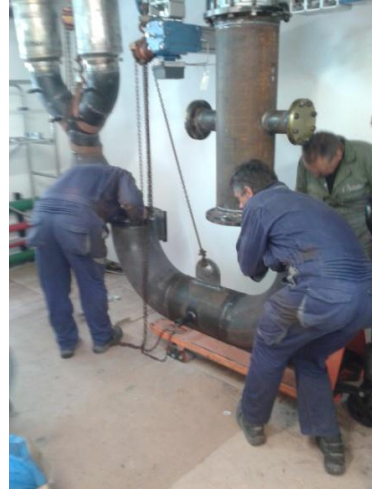
Figure 74: Installation of the lower straight part
