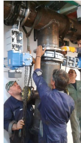
Figure 71: Installation of second butterfly valve and vertical part
