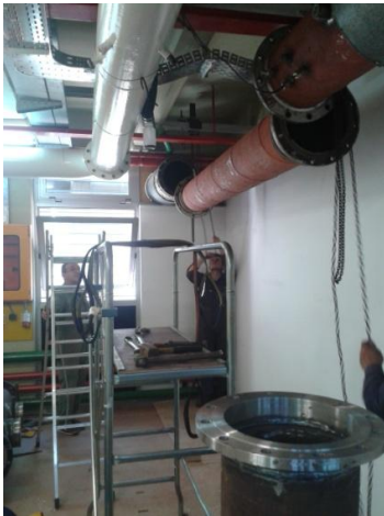
Figure 67: Removal of the previous exhaust duct
