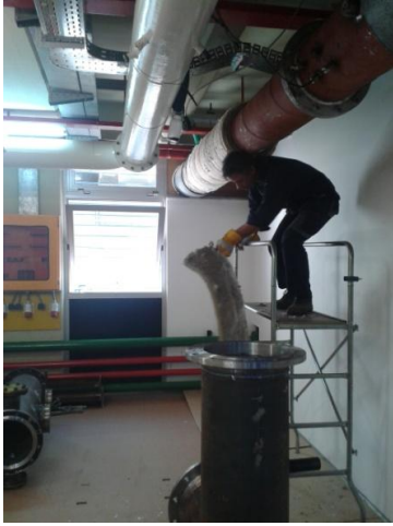
Figure 66: Removal of the insulation
