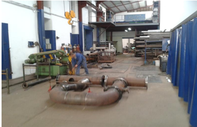
Figure 57: EBS construction in Loukis industry
