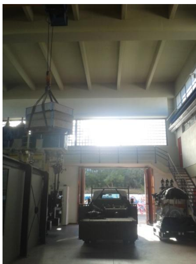
Figure 62: Butterfly valves transfer in their special boxes
