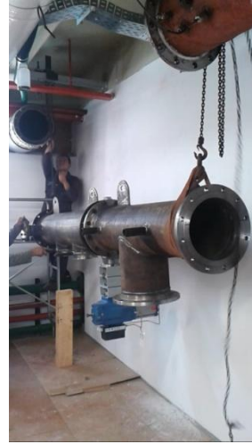
Figure 69: Lifting the assembled upper straight part
