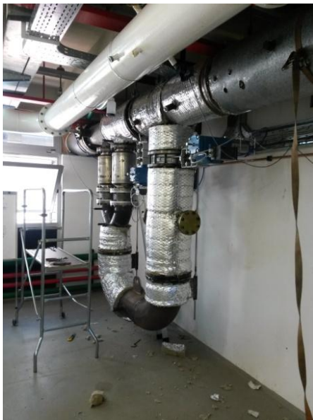
Figure 104: Installation of the exhaust pipeline insulation
