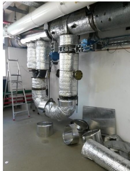
Figure 105: Placement of the insulation outer sheath (aluminium foil)
