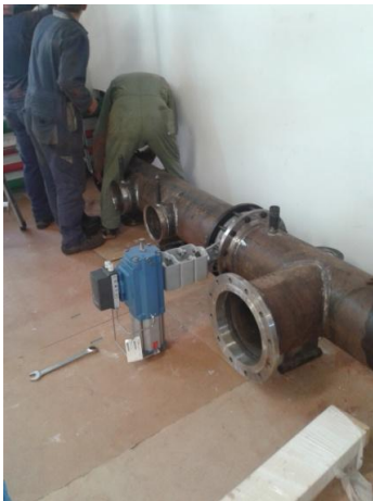
Figure 68: Assembly of the upper straight part
