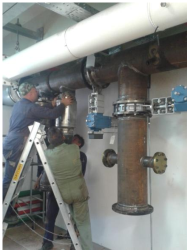
Figure 73: Lifting the DPFs part
