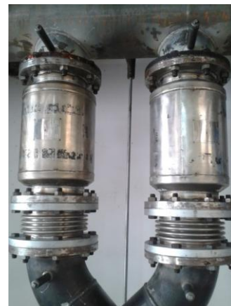
Figure 78: Flange connections and compensator
