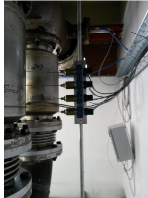
Figure 86: Pressure sensors mounted on the plate
