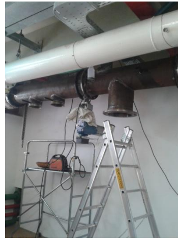
Figure 70: Installation of the straight upper part
