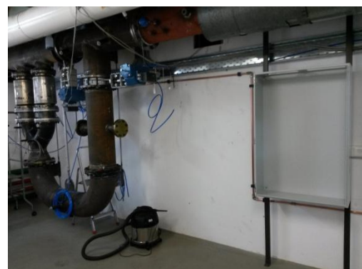
Figure 97: The panel as installed in room.13
