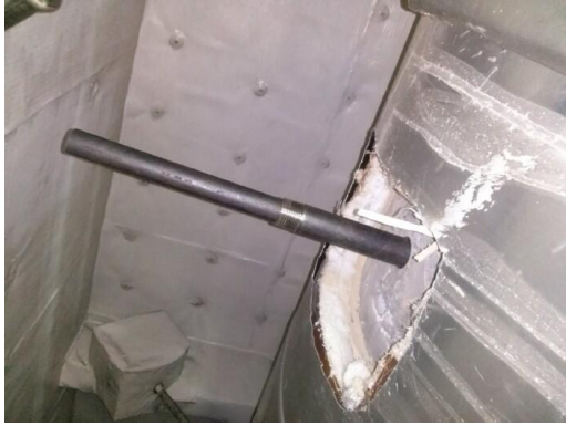
Figure 110: Guiding pipe for ensuring welding sockets alignment
