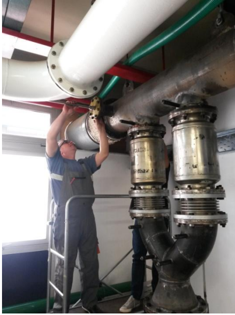
Figure 83: Inserting the pipe during alignment check
