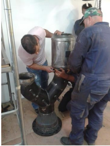
Figure 72: DPFs connection with the two-channel duct
