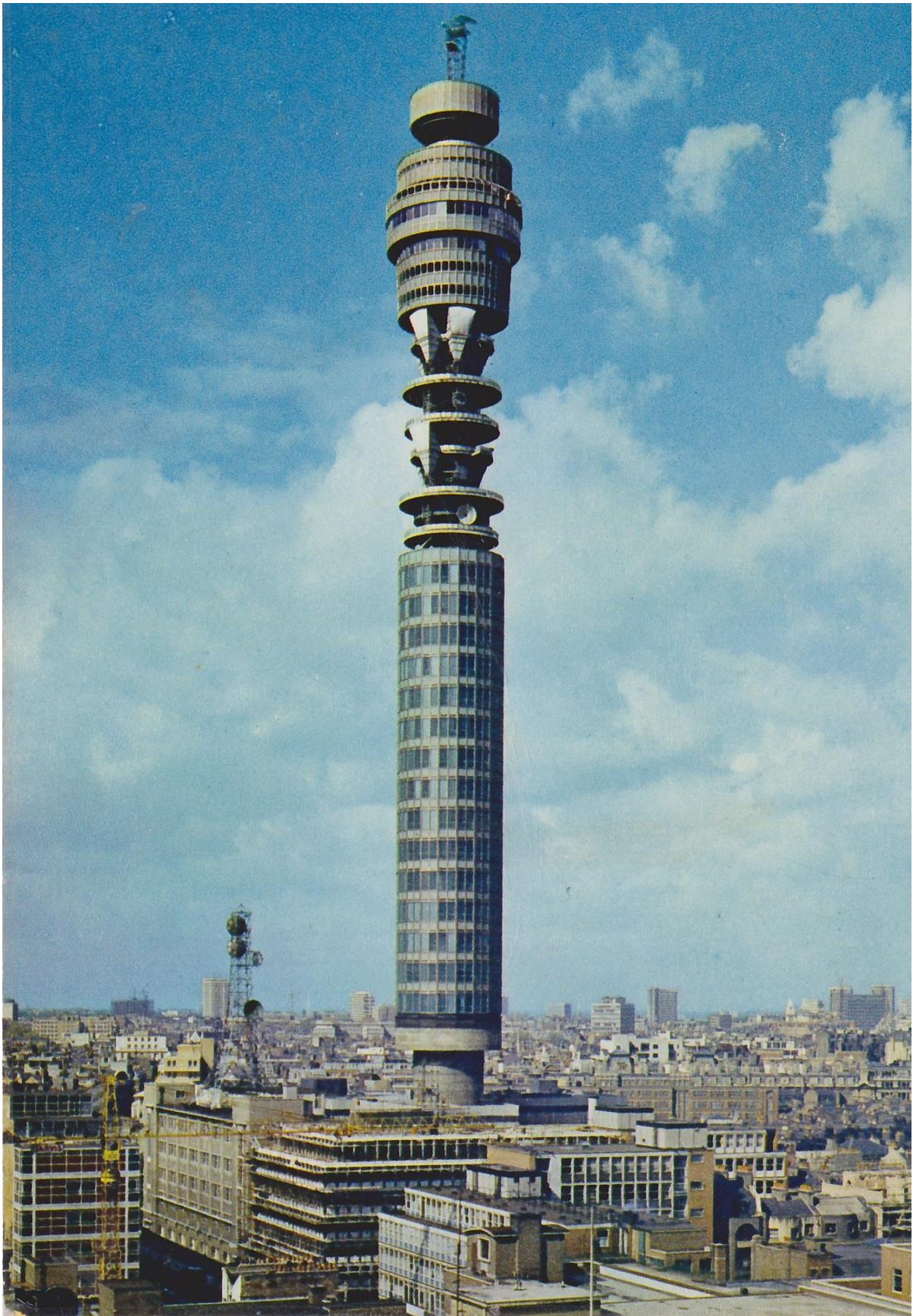
Fig. 61: Post Office Tower (2013)
