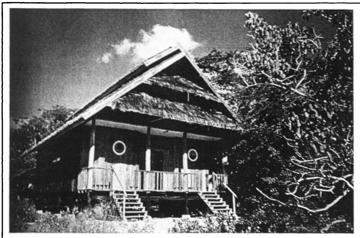
Figure 3.9 The Visitor Interpretation Building on Komodo Island.
