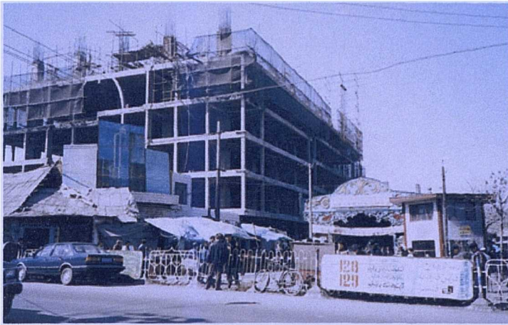
Photo 16 The entrance to Erdaoqiao market (right), dominated by a building site.
