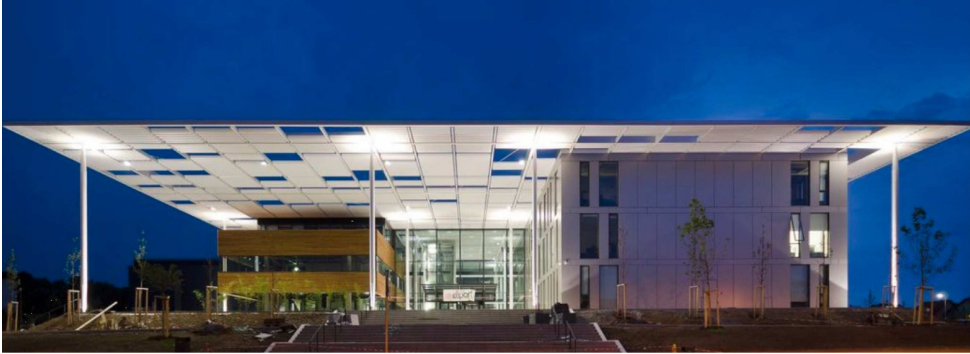
Fig. 3.12. ELI Beamlines facility in Dolni Brezany (image credit: ELI Beamlines).
