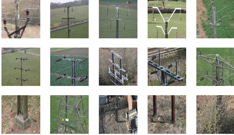
Figure 1: Top: images of S-type towers. Middle: images of T-type towers. Bottom: images from which tower type is not apparent.
