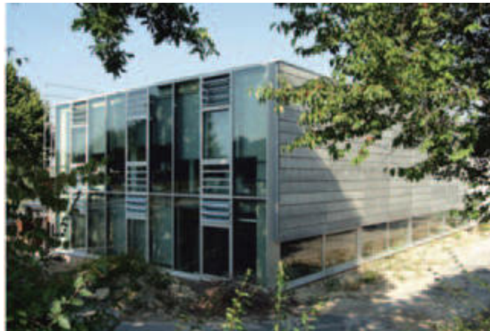
Figure 6-2: Textile reinforced concrete elements at RWTH Aachen University (Roye, Gries 2007)
