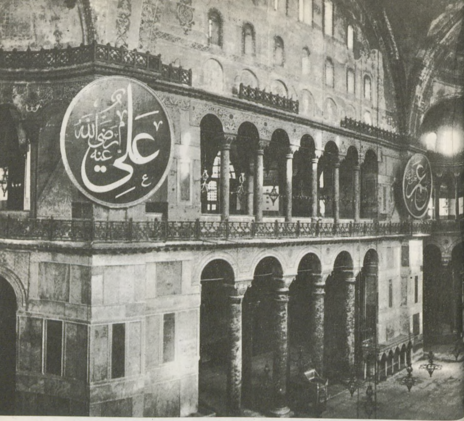
The interior of Ayasofya.
