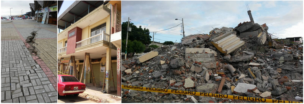
Figure 3.4: Images from personal archive showing the destruction in the coastal Ecuadorian region: (left) Caleta de Manta, seafood market in Manta city; (center) building columns reinforced with bamboo timbers in Chone city; (right) six-storey building collapsed in Portoviejo city.
