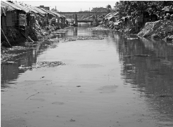
13 The canalside at Topsia
