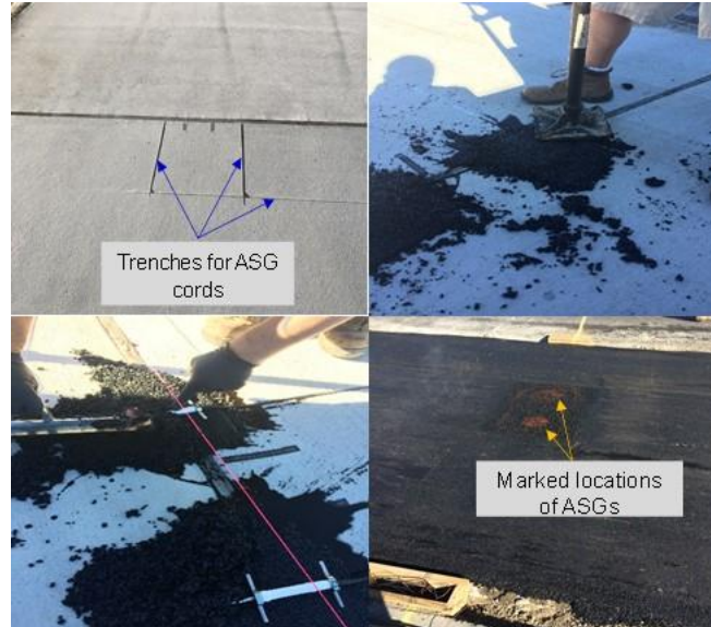
Figure 30. Asphalt strain gauge installation procedure.
