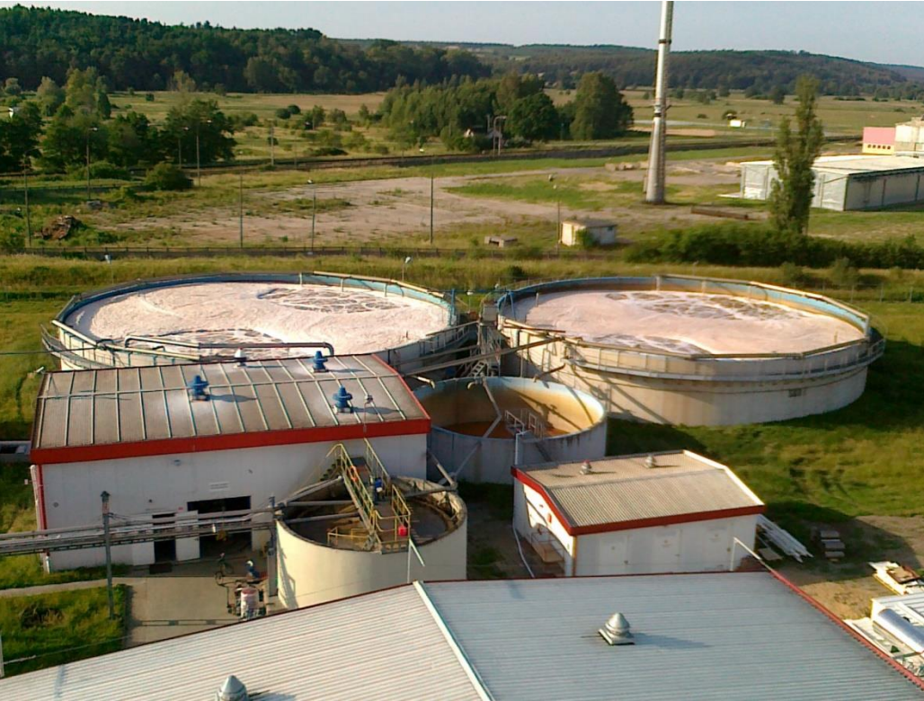
Figure 18 Aerobic stage - SBR's
