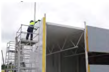
Figure 24. Sandwich panel diaphragms / www.ruukki.com/
