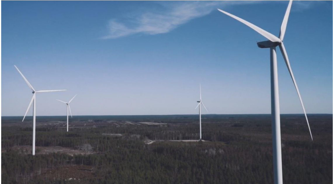
Figure 5: Horizontal axis 2,4 MW wind turbines in Honkajoki, Finland. Tower height 120m and the diameter of the rotor 117m. (Taaleritehdas, 2014)
