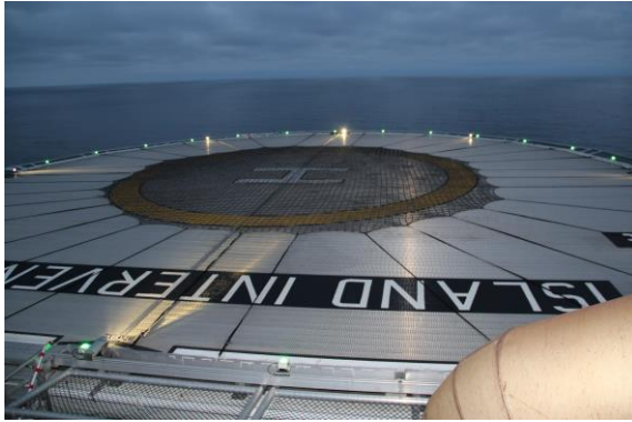
Figure 2. Helideck lighting (Picture by J. Nurminen)
