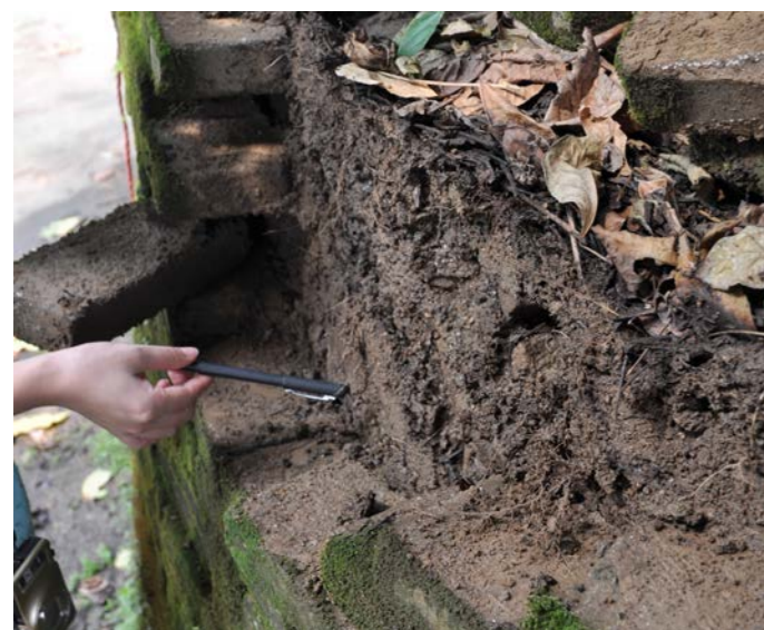
Brick wall structure containing the backfill soil
