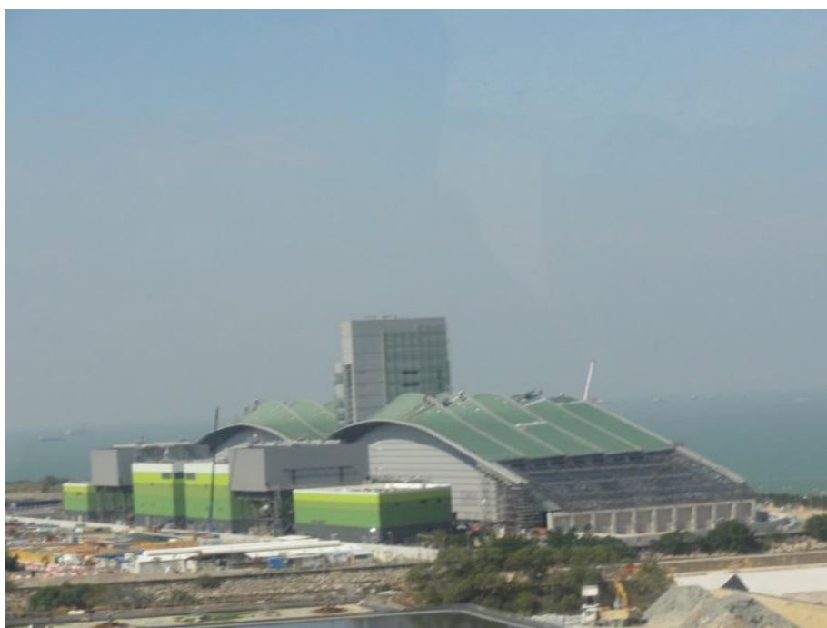
Figure 2: Sludge Treatment Facility under construction
