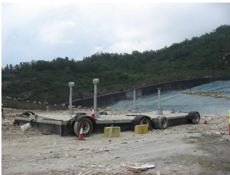
Figure 2: Cover for special waste trench
