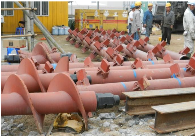
Figure 2 Auger and mixer used for pile installation
