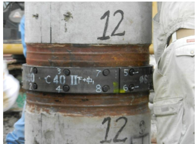
Figure 3 Mechanical splicing of PHC piles
