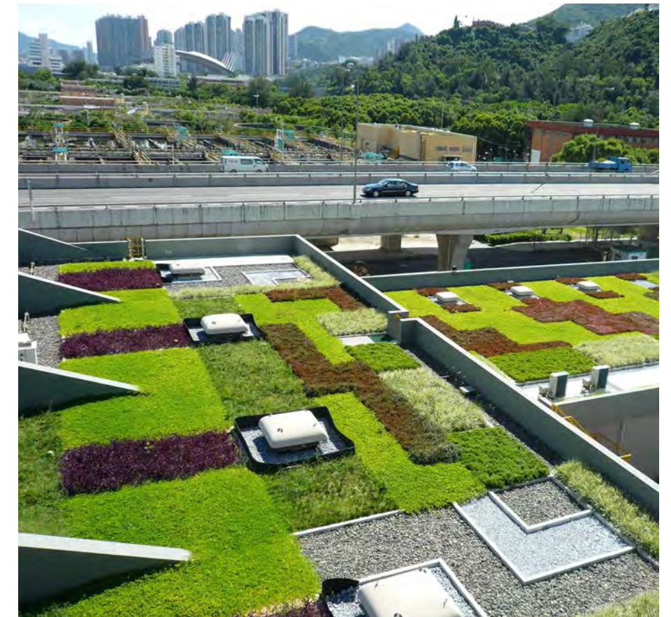
Roof greening at Sha Tin Sewage Treatment Works
