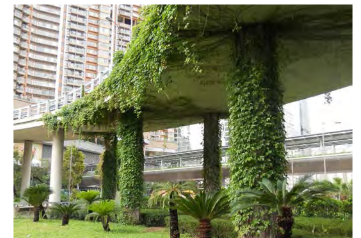
Flyover at Junction of Prince Edward Road East and Choi Hung Road
