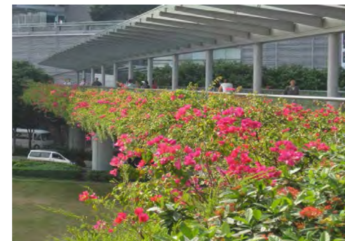
Vertical greening on IFC Footbridge
