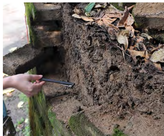
Brick wall structure containing the backfill soil
