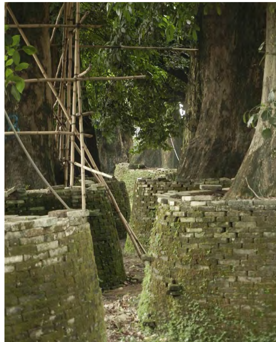
Brick walls built to create a new root ball
