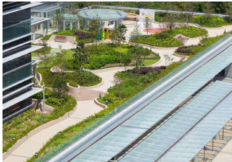
North Lantau Hospital (Source: Architectural Service Department)
