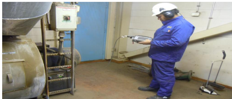
Figure 5 Vibration measurement being performed in the field.
