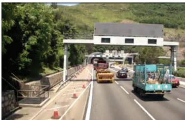
(B1) Entrance to the Cheung Tsing Tunnel is surrounded by green vegetation on both sides
