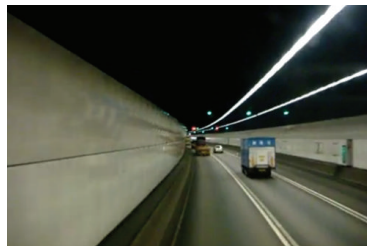
(B2) The 1.6 km long Cheung Tsing Tunnel is equipped with jet-fan longitudinal ventilation
