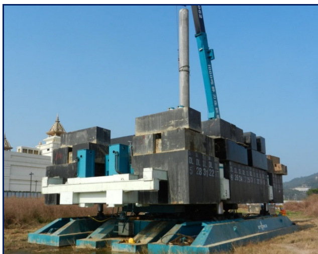
Figure 2: Pile jacking machine for PHC piles
