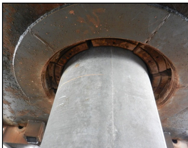
Figure 3: Clamping of PHC pile
