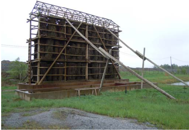
FIGURE 1. Willow stack tower in Vaasa
