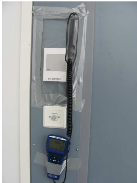
Figure 9. Installation of “bag” comparing of sensors
