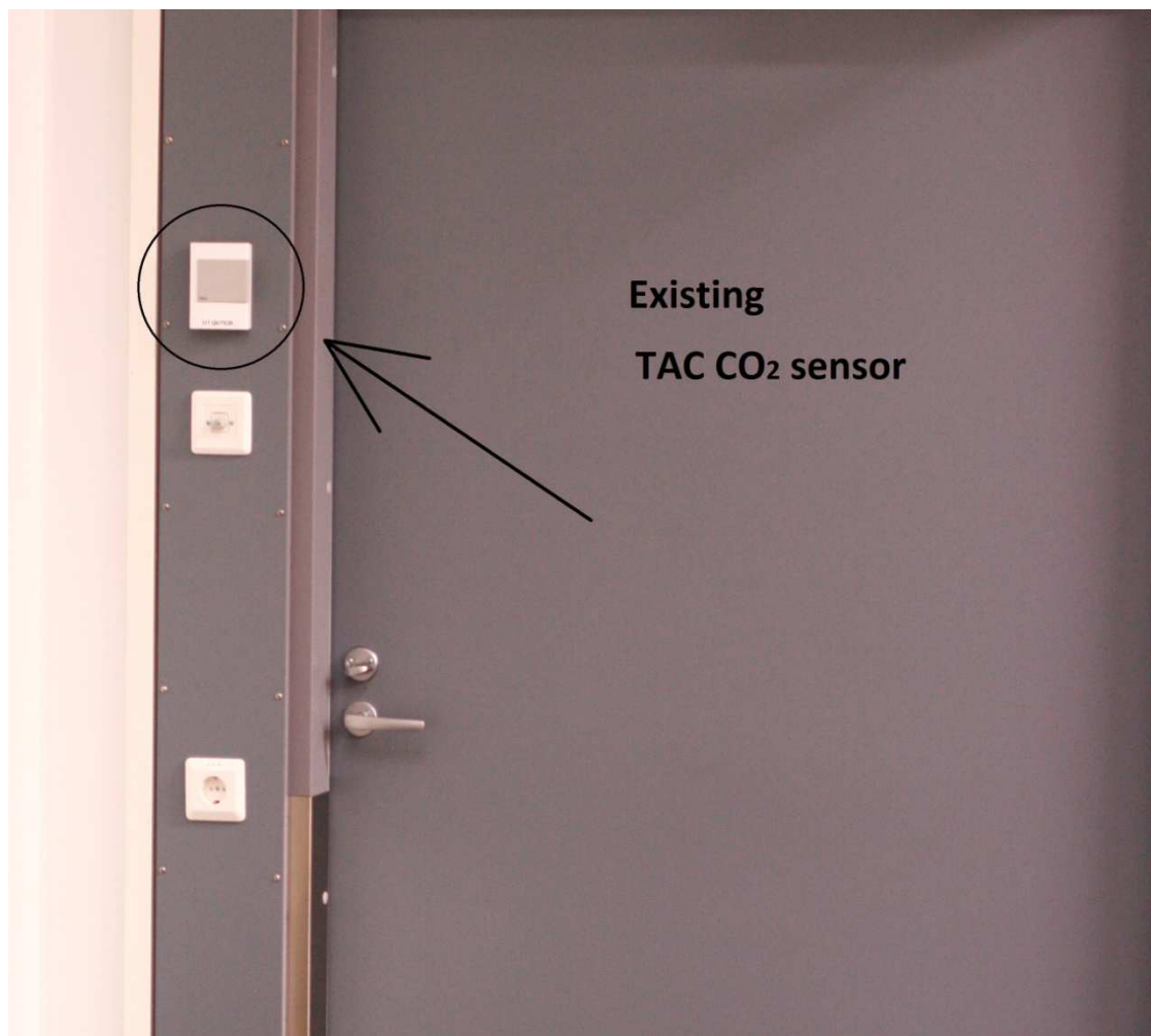
Fig.7 Current location of system's carbon dioxide sensor
