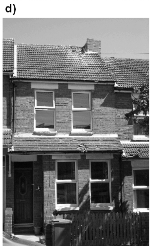
Figure 7. (a) Damaged chimneystack and secondary damage to roof tiles, (b) Cracks in brickwork (Radnor Park Road), (c) Cracks extending through the roof line of a building at Grace Hill, (d) Collapse of chimney stack to roof level and associated roof damage (Stuart Road), and (e) Marshall Street: 1930's style terraced houses with relatively high density damage.
