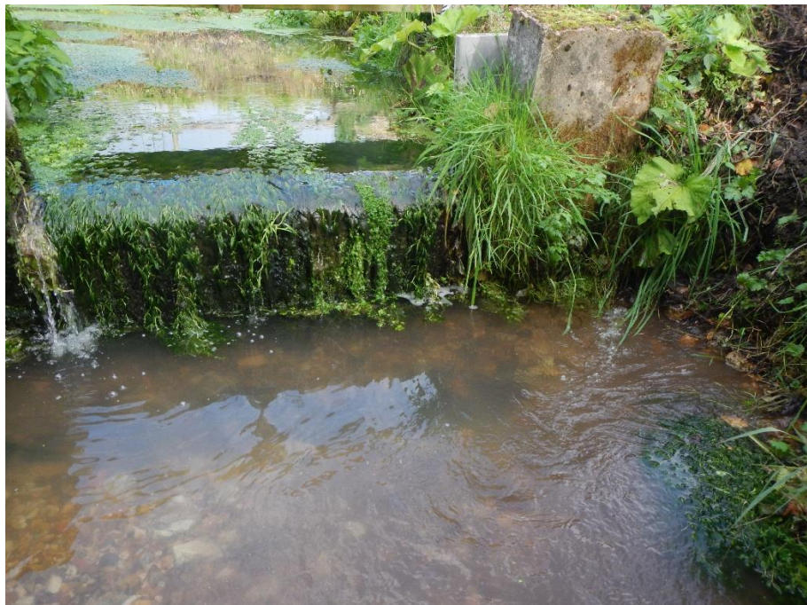
Figure 31 Turbid water below the discharge weir on The River Crane in autumn 2017 following watercress bed cleaning operations. The outflow is much reduced to limit sediment release, but suspended solids still entered the river at CRDS1, where levels at 8.5mg/L were recorded downstream
