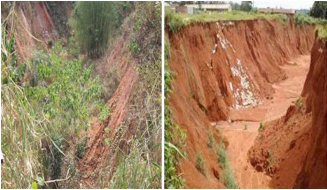
Figure 31: Revegetating and Active paths of Iyoku Gully site
