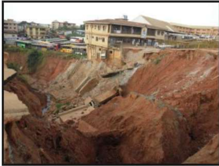
Figure 1:Gully Erosion in Onitsha southeast Nigeria
