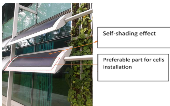
Figure 3.13 Self-shading effect and preferable installation of PV cells according to Hwang et al. (2012), Kang et al. (2012), and Yoo & Lee (2002).
