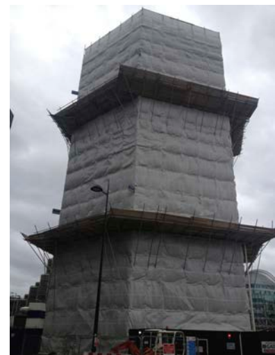
Figure 118: Covered scaffolding near Victoria Station, London, 2013.
