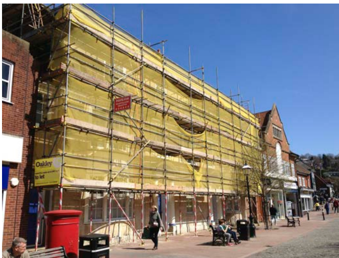
Figure 117: Covered scaffolding, Lewes, UK, 2013.
